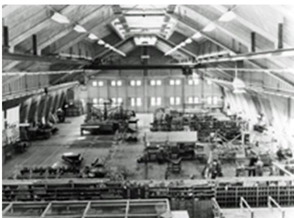
Nitarbeten i Monteringshallen (By 6)
